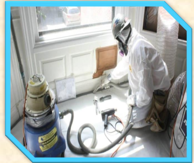
A removal agent in proper PPE
