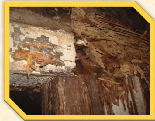
Termite damage
