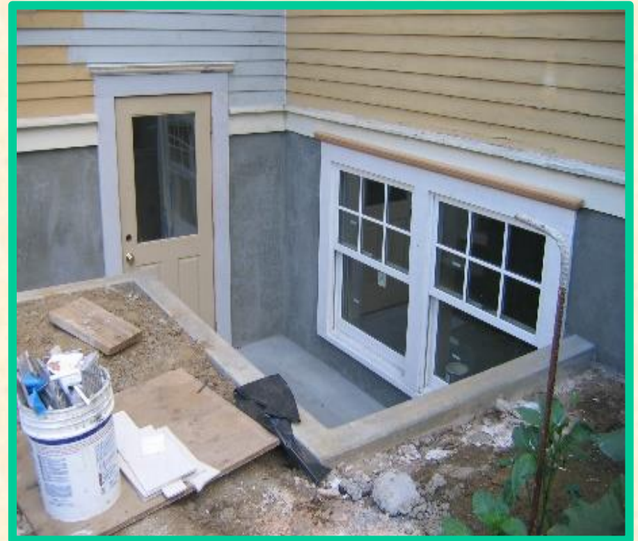
Below grade windows under construction
